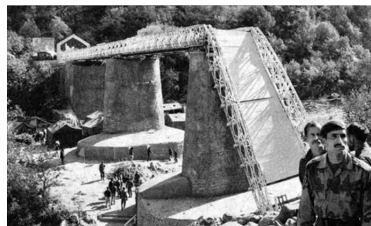
Figure 3.15: A view of the damaged Aman Setu at the LOC in Uri, due to an earthquake
